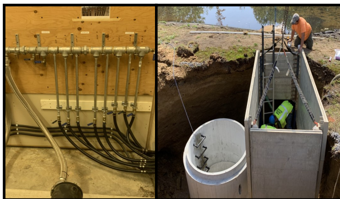
Air Distributor Mods/Installing Pump Station
