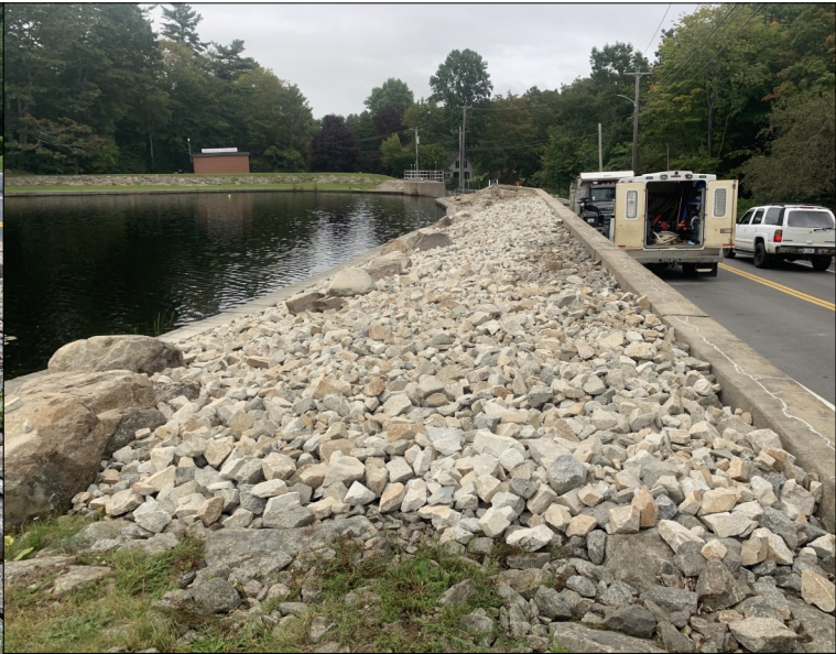
After rip rap was removed
