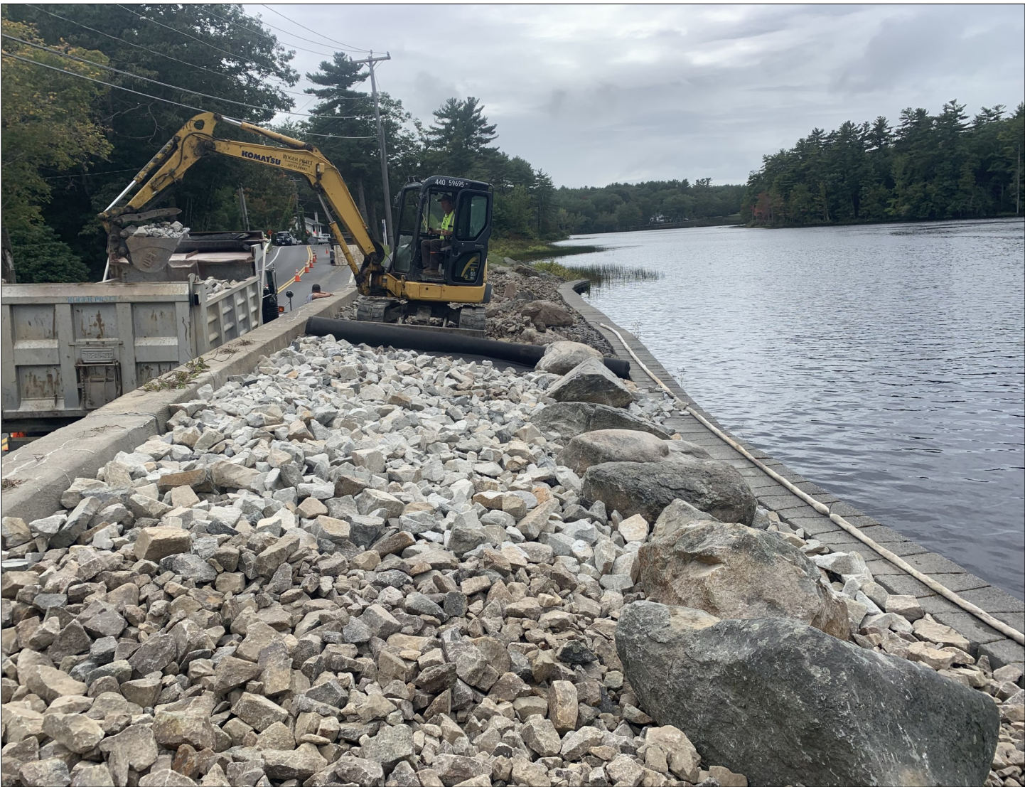
Roger Pratt replacing rip rap on the dam
